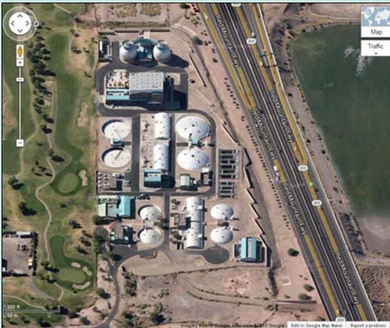
Mesa Northwest Water Reclamation Plant
