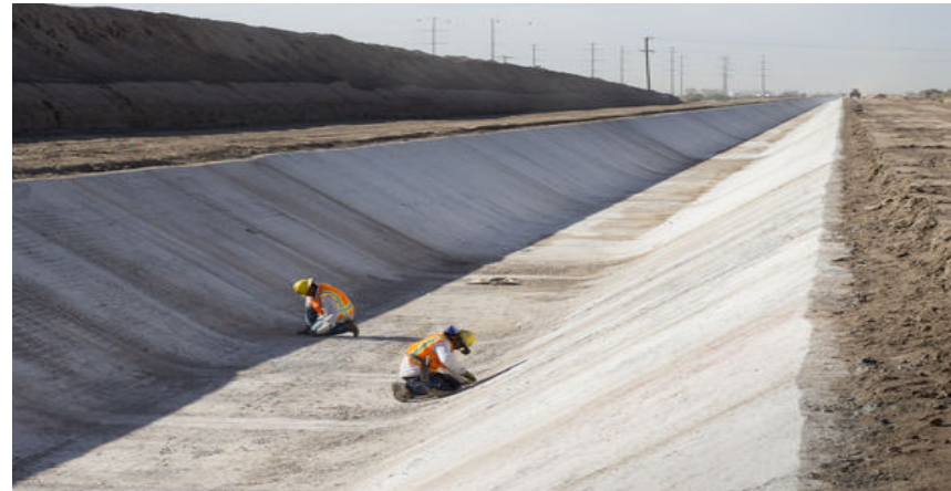
Construction work continues on the concrete lining of the Southside canal.
